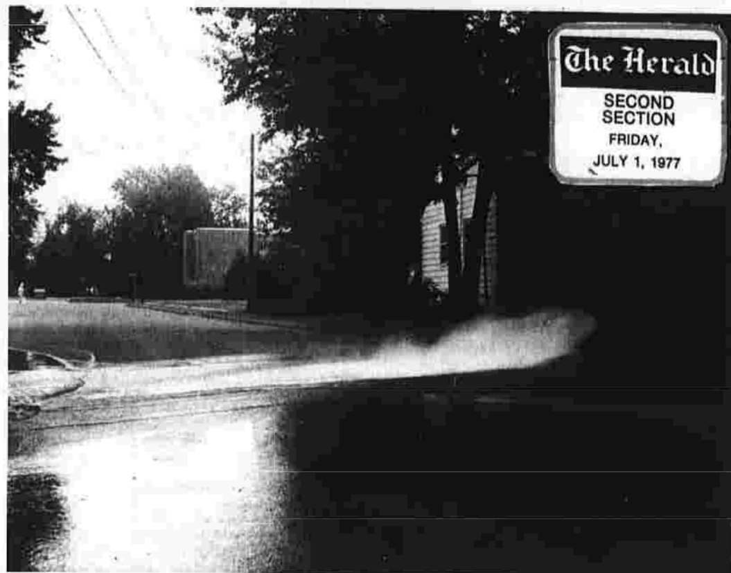
Water main being flushed
